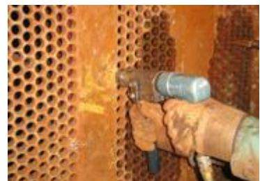
**Step 3** The 3rd step is to pull the tube on the opposite end. It is pulled about 4 inches from the face of the tube sheet with the pulling system, than the whole tube is pulled manually.
