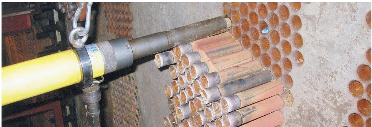
**Step 4** The 4th step is to pull the stubs from the tube sheets left in place from the first step.
